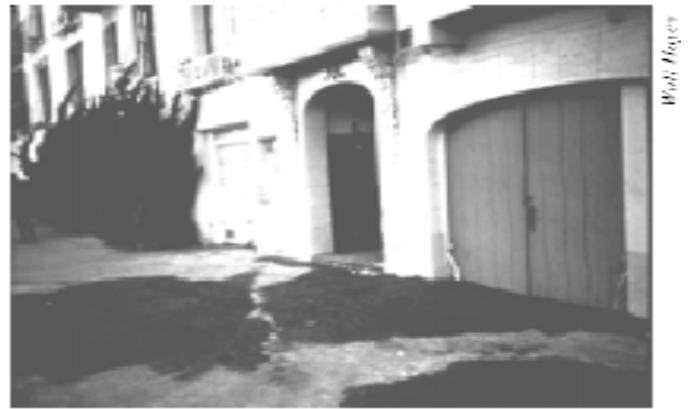
Figure 40 - Loma Prieta Earthquake, October 17, 1989. Lateral spreading, liquefaction and sand boils caused extensive damage in the Marina District of San Francisco, about 60 miles away from the epicenter.
