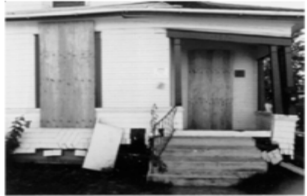
Figure 13 - This home wasn't bolted and slid off its foundation. Sometimes the damage can be so bad that houses have to be demolished.
