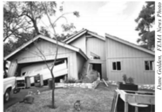
Figure 5 - San Simeon Earthquake, Dec. 22, 2003 This home slid two feet off its foundation due to inadequate nailing of walls to its sill plates.
