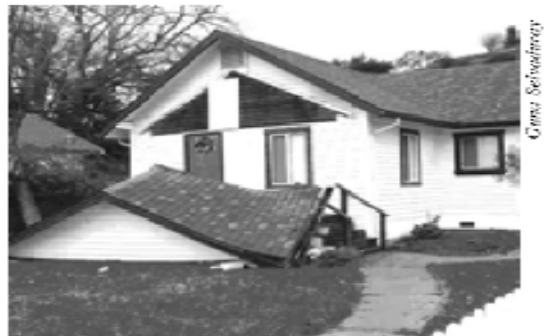
Figure 6 - San Simeon Earthquake, Dec. 22, 2003 The collapsed porch was not adequately attached to this single family residence.
