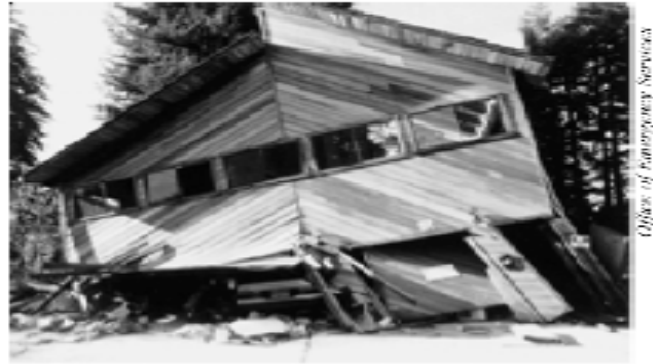
Figure 29 - This mountain home was built over a garage, and its walls were not strong enough to withstand an earthquake.
