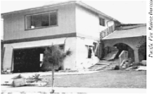
Figure 1 - San Fernando Earthquake, Feb. 9, 1971 Severely damaged split level 1 and 2 story wood frame dwelling. The one story portion dropped about 3 feet.
