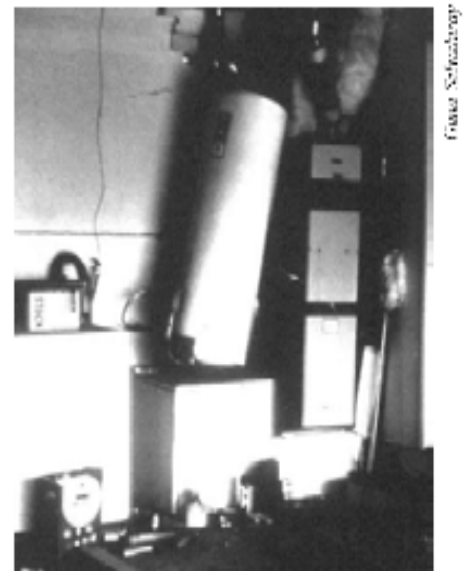
Figure 11 - This unstrapped water heater tipped over during the 1984 Morgan Hill Earthquake. Fortunately gas and water lines were not ruptured
