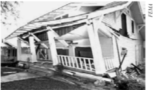
Figure 3 - Northridge Earthquake, Jan. 17, 1994 Single family residence damaged due to failure of multiple elements.
