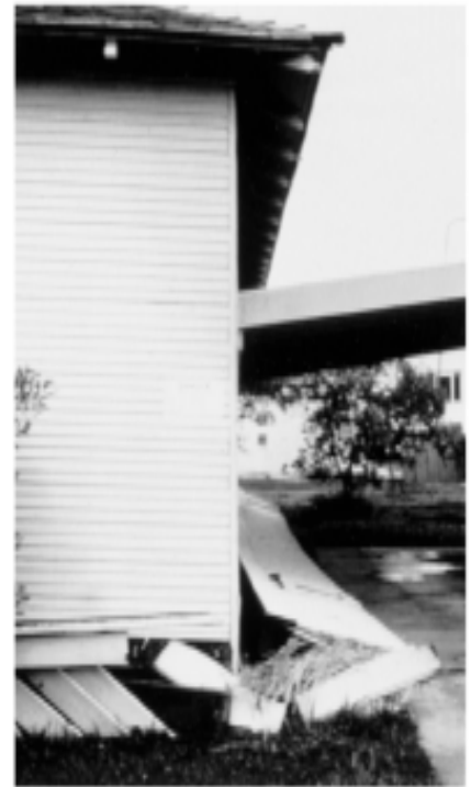
Figure 15 - Damage to home due to cripple wall failure.
