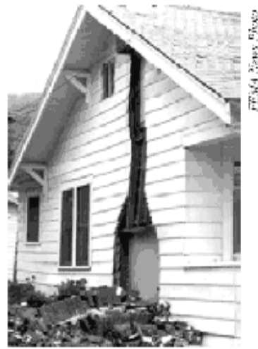
Figure 4 -Northridge Earthquake, Jan. 17, 1994 Chimney Collapse - common type of damage to unreinforced masonry.
